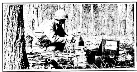
GAS GUN -- SP4 Roger Brooks of Elizabethtown checks out a machine gun simulator during field training exercises during last weekend's drill. The device utilizes liquid propane gas and a spark plug to simulate the sound of an M-60 machine gun. Assigned to the 35th Aviation Brigade of Frankfort, Brooks said, "The training that we are doing today is as good as (that which) we get overseas." (Photo by SSG Ron Bayes, 133rd PAD)
